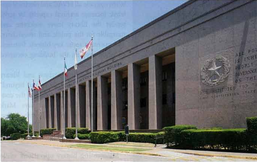
Harvey-Cleary's CM-at-risk contract for the renovation of the archives and library building (shown, exterior) allowed the firm to coordinate early with the Texas Facilities Commission. Photo: Bailey Architects.
